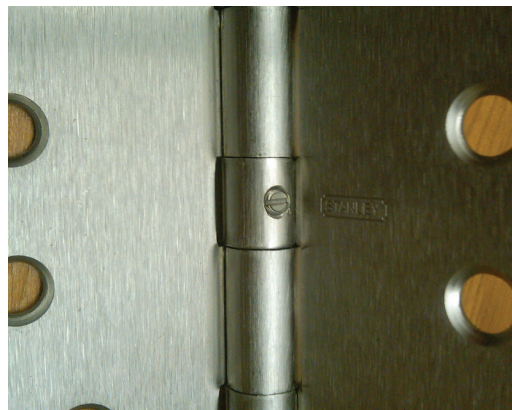
Figure 4. Non-removable pin hinges should always be used on any perimeter door that swings out, particularly on the backside of commercial buildings and on doors opening out into desolate areas.
