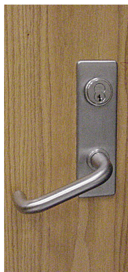
Figure 5. This lever set was attacked and deformed; however, it still functions.
