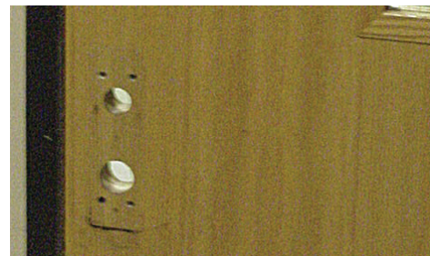
Figure 4. When a vandal deforms a door and/or its locking hardware, intended egress might be negated. In this case, the vandalized door certainly will not prevent egress.
