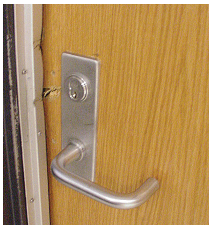
Figures 1 and 2. Vandals attempted to separate the door and its lever set from the frame by pounding and prying (left). To alleviate the effects, a simple one-inch cover plate was screwed into the door to cover the holes (right).
