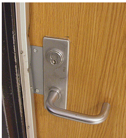
Figures 1 and 2. Vandals attempted to separate the door and its lever set from the frame by pounding and prying (left). To alleviate the effects, a simple one-inch cover plate was screwed into the door to cover the holes (right).
