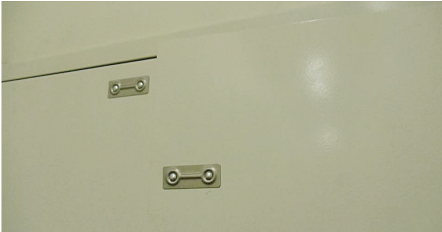
Figure 5. The upper and lower latches use a plate on the outside of the door.
