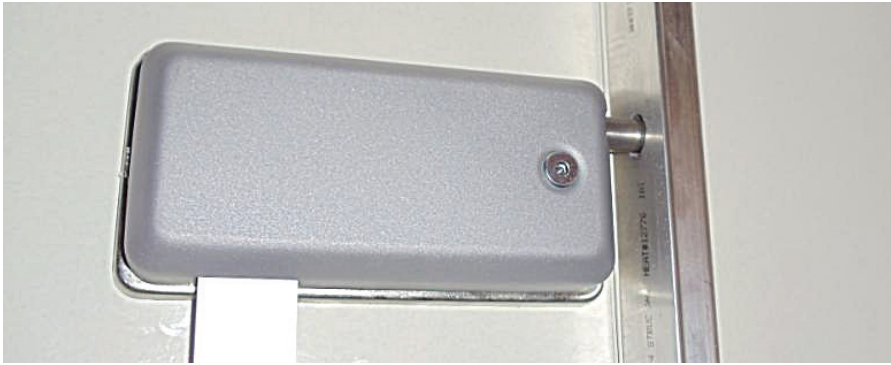
Figure 7. Notice the latch bolt going through the angle.
