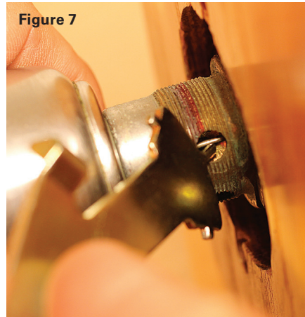
Figure 4. Here's what you'd see if you looked behind the rosette while turning the inside knob, if installed on a door. In the following pictures, I've removed the rosette so you can see what I'm doing more clearly. In practice, you wouldn't be able to remove the rosettes without removing the knobs.
