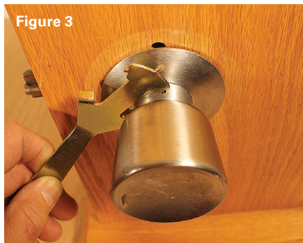
Figure 3. Here, you can see the lock mounted in a display and a spanner wrench being used to loosen the inside rosette. The lock is held in place by tightening the rosettes instead of using screws. Spin the rosette back toward the knob as far as you can.
