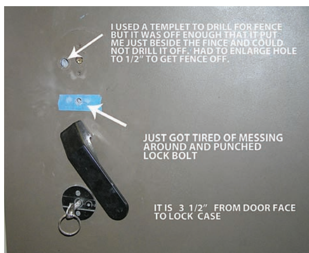
Figure 7. The author punched the lock bolt out of the way and opened the door.
