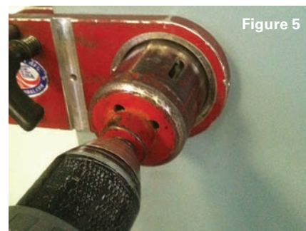
Figure 5. Here, the hole saw is in use. This is the most likely place for you to hurt yourself and the door. You don't have a pilot hole to stabilize the saw, so take your time, and make sure the jig doesn't move. Keep a tight grip on the drill, as the saw is likely to jam against the old hole's edge as it cuts.
