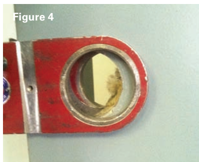
Figure 4. This image shows a boring jig placed over the hole and lined up with the bolt hole on the door's edge. Make sure the jig is as tight as it can possibly be. The 2½" hole looks slightly off because it is. The previous install was a little inaccurate, but I'll fix that shortly.
