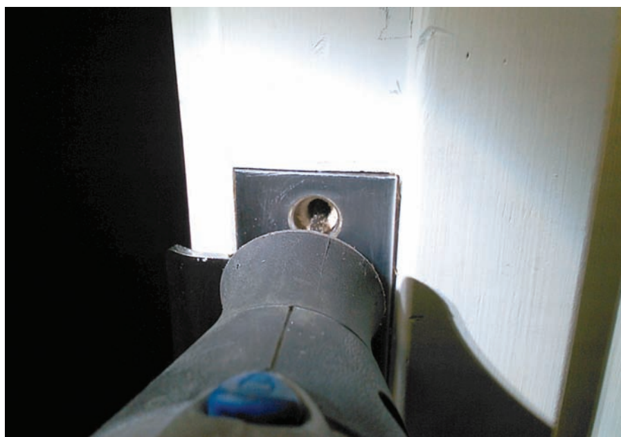
Figures 2 and 3. Carefully put the tip of the tool bit against the broken screw, turn on the Dremel tool, and grind out the broken screw.
