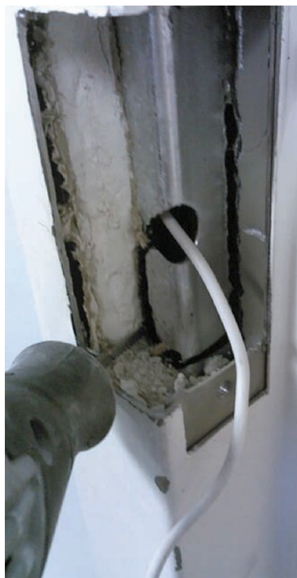
Figures 8 and 9. It takes about three to four minutes to cut out the sheet rock and metal stud.
