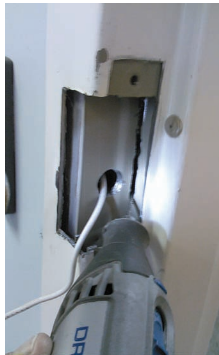
Figure 7. Walk the bit around the door frame's inside to make the necessary cutout.
