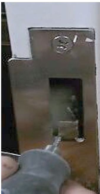
Figures 4 and 5. Carefully cut along the marker line to extend or modify the latch hole. Marking and cutout takes about two minutes to complete, with no filing.
