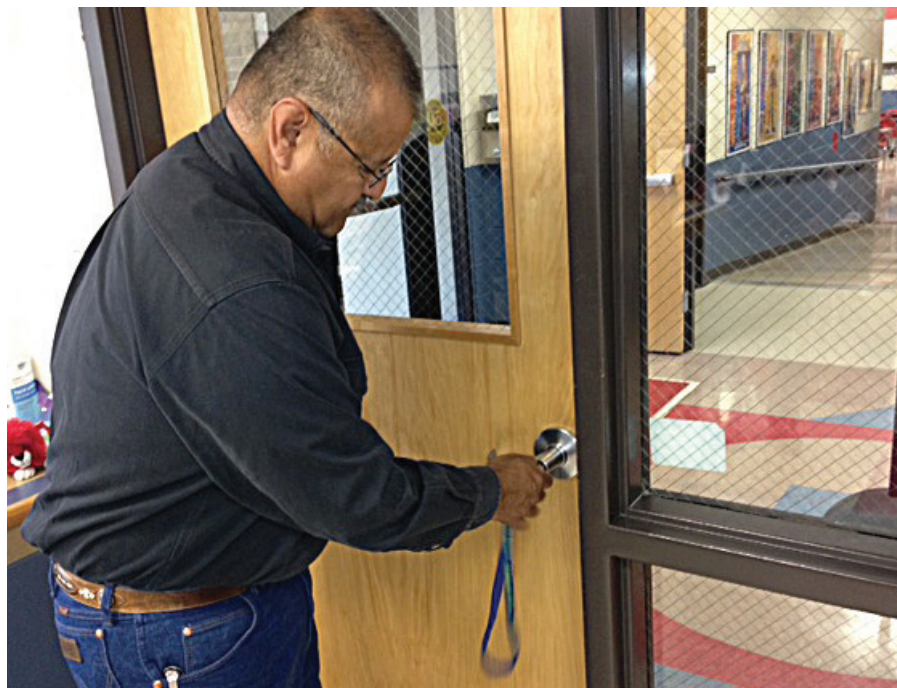
Vince Flores, building trades manager of maintenance and operations for the Northside Independent School District in San Antonio, TX, demonstrates the use of the intruder lock function on one of the classroom doors at Locke Hill Elementary School.
