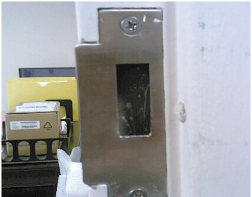
Figures 4 and 5. Carefully cut along the marker line to extend or modify the latch hole. Marking and cutout takes about two minutes to complete, with no filing.
