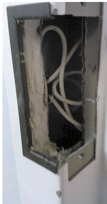
Figures 8 and 9. It takes about three to four minutes to cut out the sheet rock and metal stud.
