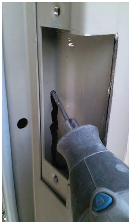
Figure 6. Push the bit to drill through the metal and start cutting.
