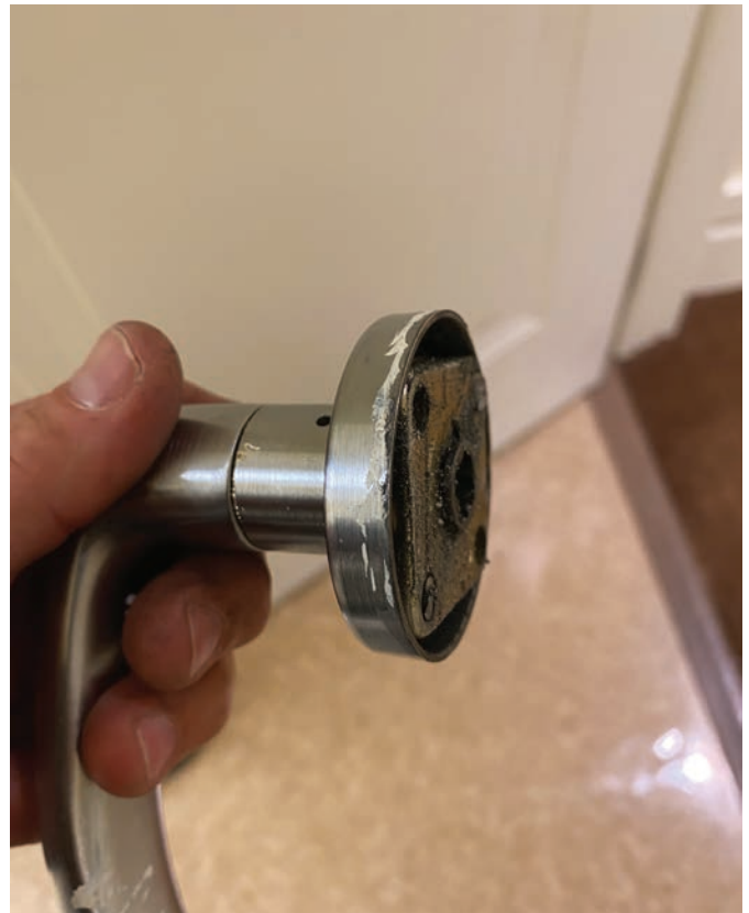
Figure 2. The author Sawzalled off the inside lever.
