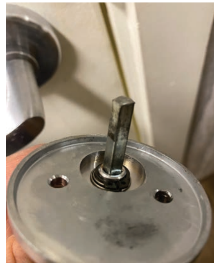
Figure 11. The thumbturn spindle extended into the lock so far that it needed to be shortened so the emergency key would fit.
