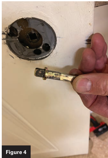
Figures 4 and 5. The Schlage spindles were undamaged and fit neatly into the BEST levers.
