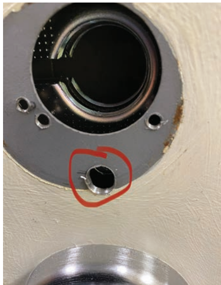
Figure 9. This is what the author saw when he took off the outside plate on a bathroom door. He added the hole.
