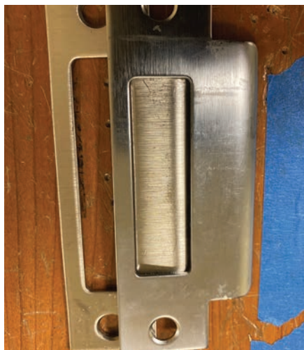
Figure 12. It's important to change out the strike plate when retrofitting and to op-check the installation before you walk away from it.
