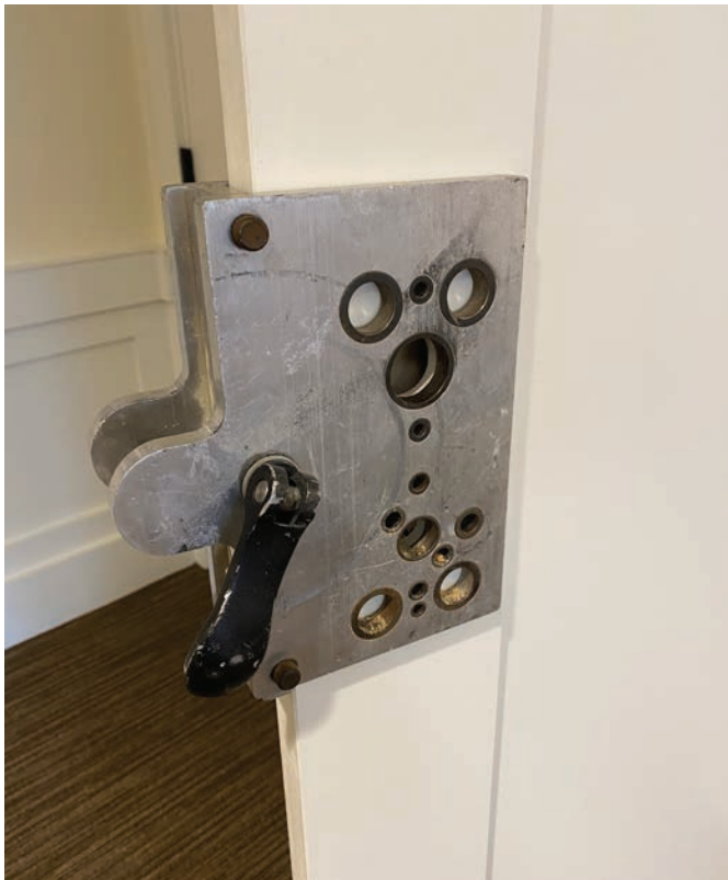
Figure 1. The old prep was missing two holes required for the 45H, so the author used a BEST jig to drill them.
