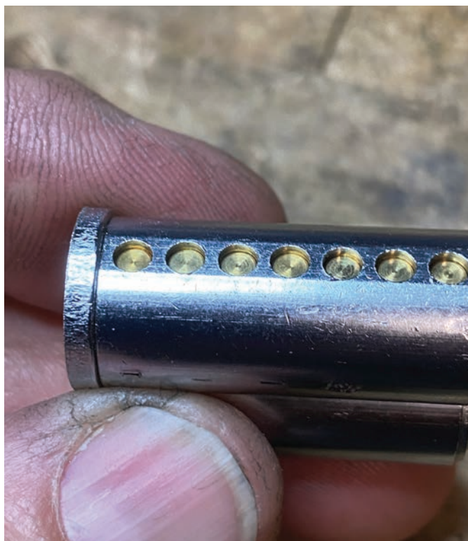
Figure 20. Tilt the core, and you'll notice that the pins in every chamber are the same height.
