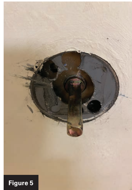
Figures 4 and 5. The Schlage spindles were undamaged and fit neatly into the BEST levers.
