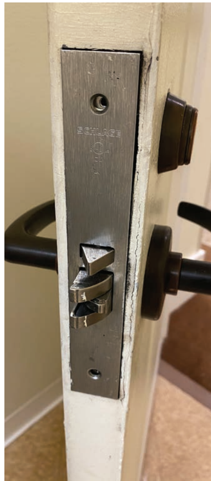
Figure 8. The job is complete, minus the faceplate screws.
