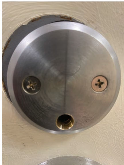
Figure 10. The installation crew lined up and drilled a hole through the blank plate and reused it.
