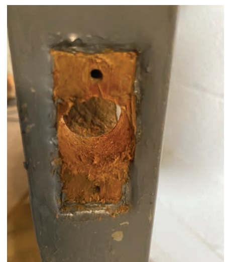
Figure 14. The latch mortise needs to be enlarged for the larger backset.
