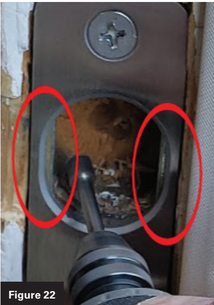
Figure 19. The author added a strike reinforcement plate.
