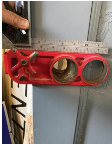
Figure 10. The Kwikset jig clamped onto one of the Kalamein doors.
