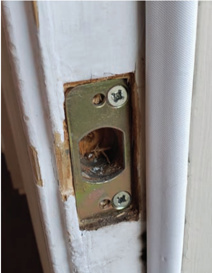
Figure 19. The author added a strike reinforcement plate.
