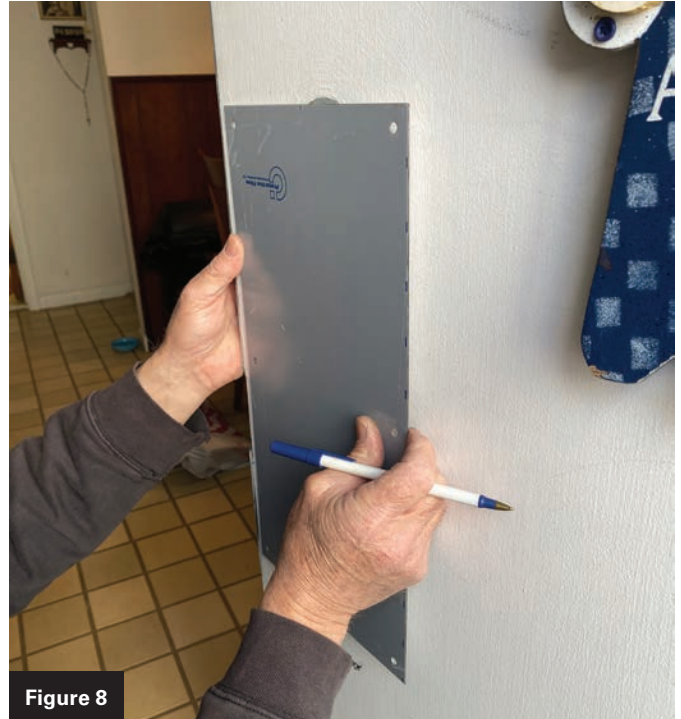
Figures 7 and 8. Here you can see what had to be covered and the 8" x 16" plate used to do it.
