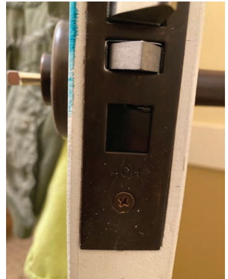
Figure 26. This finished fix neatly conceals the rocker.
