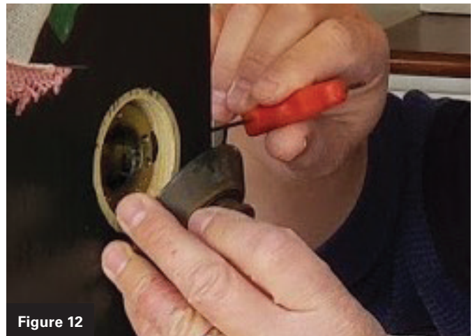
Figures 11 and 12. The screw is located under the faceplate of the bolt, and a long \frac{5}{64} " Allen wrench is required to reach it.
