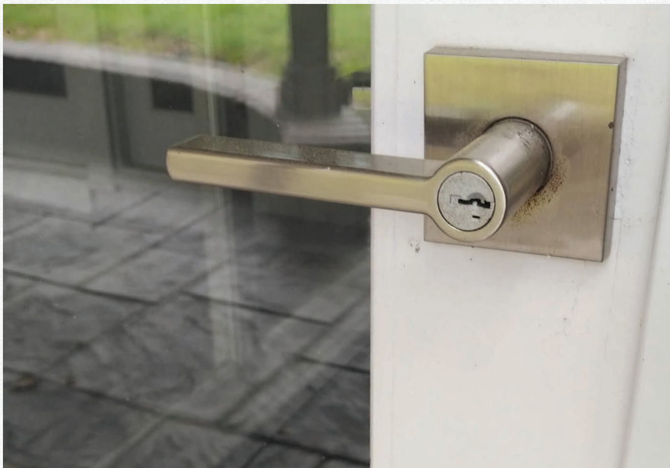
Figure 6. Eleven of these would have been tremendously wasteful and expensive to drill and replace, but the LockTech decoder and tryout keys had them all reset in a matter of minutes.
