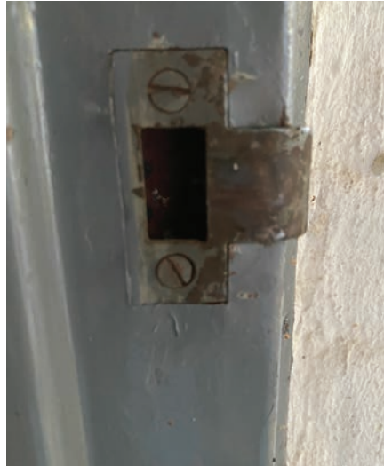
Figure 16. The existing strike had to be used because it was a lot smaller than a standard strike.
