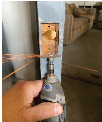
Figure 19. A Dremel was used to help center the latch.
