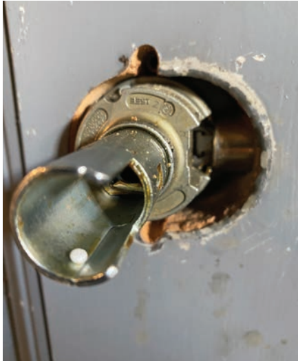
Figure 15. The author cuts the holes into the “U” shape seen here because the holes tend to be tight.
