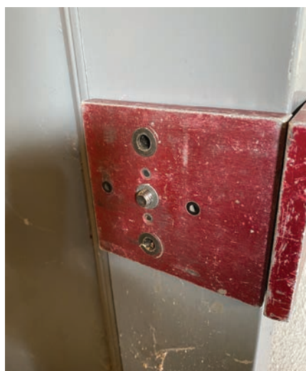
Figure 13. The author likes to use this Major jig for the \frac{5}{16} " holes for the studs.
