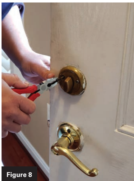
Figures 7 and 8. The author used Vampire pliers to get the stripped screw out.
