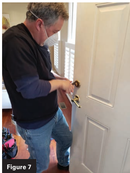
Figures 7 and 8. The author used Vampire pliers to get the stripped screw out.
