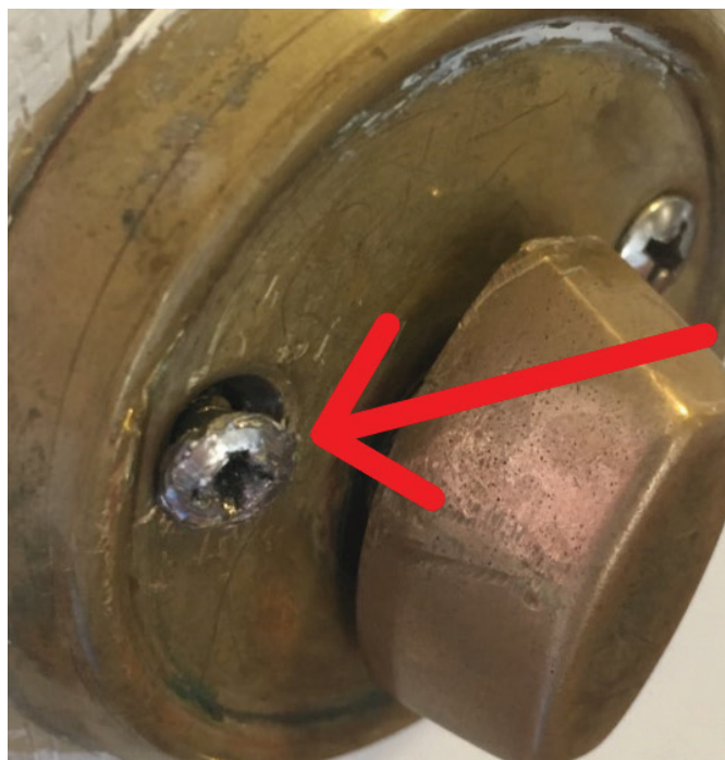
Figure 2. One of the screws holding the lock to the door was stuck and wouldn't go back into the lock.
