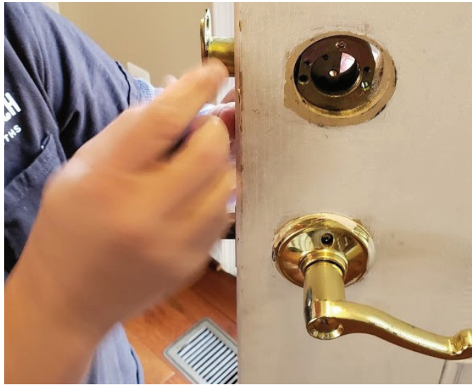
Figure 13. The author removed the existing Lori deadbolt.
