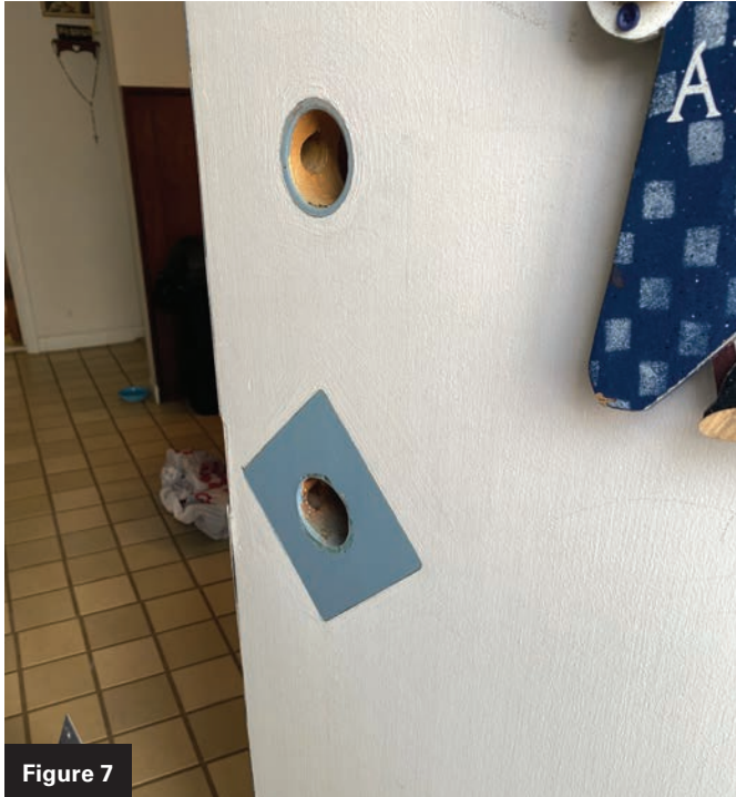
Figures 7 and 8. Here you can see what had to be covered and the 8" x 16" plate used to do it.
