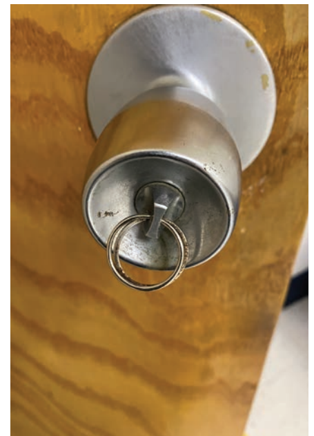
Figure 5. Here's an interesting way to get a better grip on a cylindrical thumbturn.
