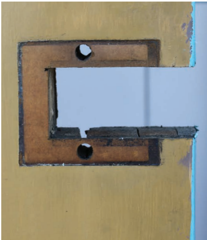
Figure 3. The lock prep is a square cutout with the addition of the two through-bolt holes.
