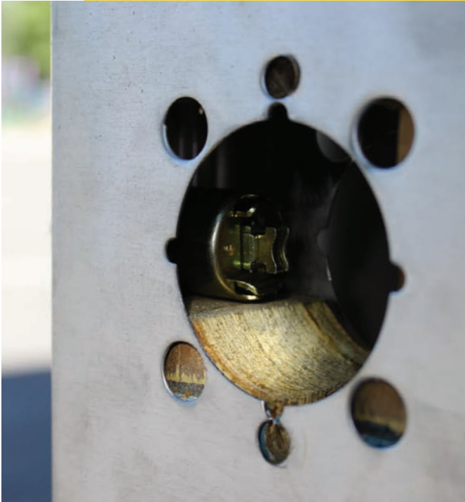
Figure 9. The biggest issue I have with using just a wraparound plate is the lack of support for the latch at the retractor. Over the years, the latch disconnected from the retractor from someone yanking hard on the door.
