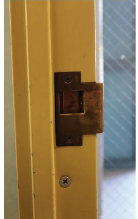
Figure 6. Keep in mind that the locks and strikes are handed. This one has the opening to the top instead of the bottom like the last one.
