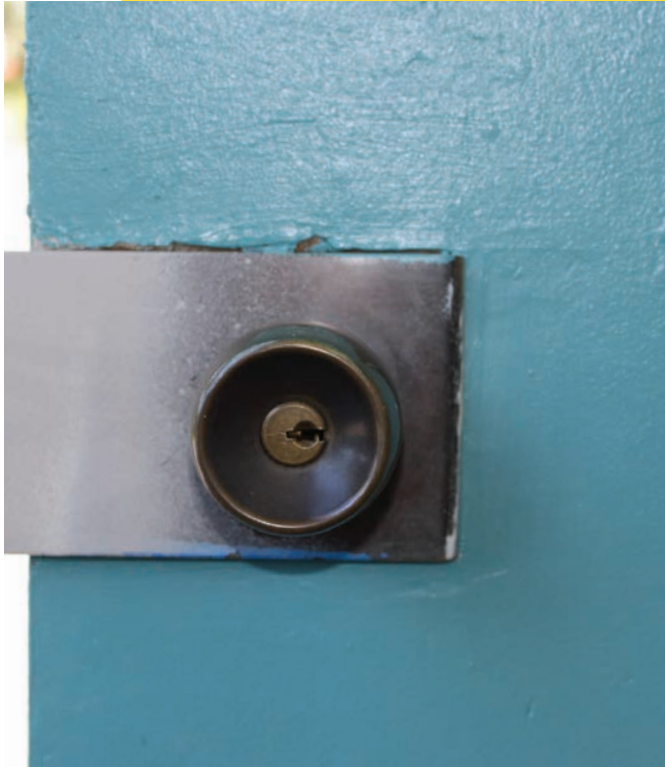
Figure 1. The outside of the Unit lock is shown. It has a nice look and includes a latch guard.
