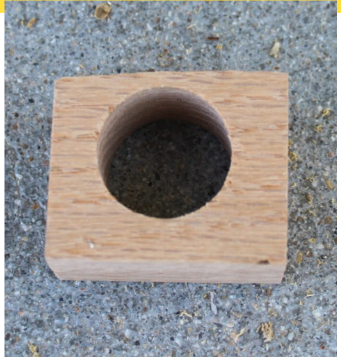
Figure 10. This is a shop-made block to support the latch. It's made from \frac{3}{4} " stock and cut to match the door thickness. In this case, 1\frac{3}{4} "; other times, they are cut to fit inside a hollow metal door to support the latch.
