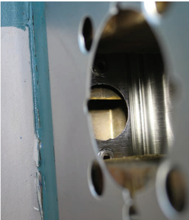
Figure 7. We dropped the plate a little to align the latch to the strike opening. Notice an issue with the cross bore?
