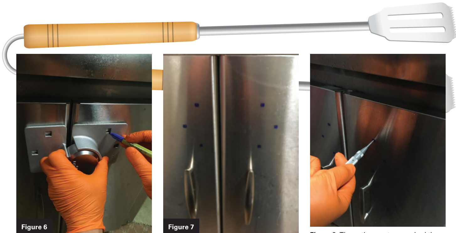
Figure 8. The author center-punched the holes that he marked.
