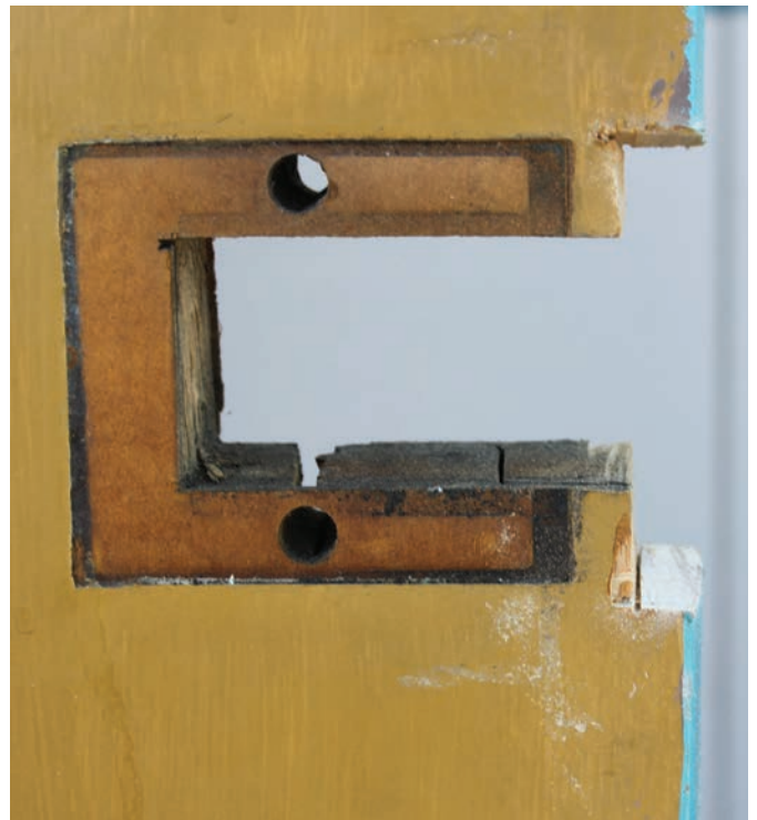
Figure 4. The wraparound plate latch support is too tall to match the existing cutout. This requires cutting or notching the top and bottom of the cutout.
