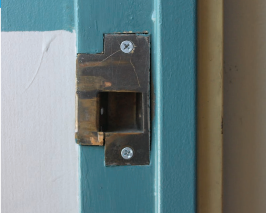
Figure 5. The next challenge we faced was the strike. The Unit lock uses a 3¼" tall strike with an offset cutout. Compare this to the common T strike, which is only 2¾" tall with a centered opening. We looked at making new strikes but decided to keep the old ones and line the latch up to the opening in the strike.
