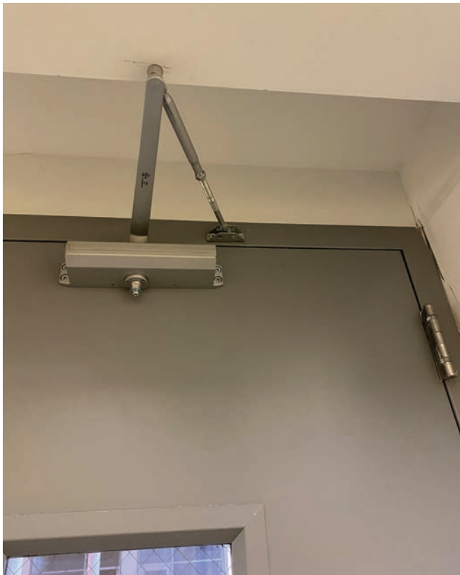
Figure 1. The closer is installed backwards.
