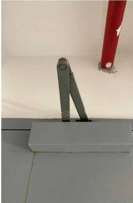
Figure 12. The author was able to move the arm to the right and preload it a bit.
