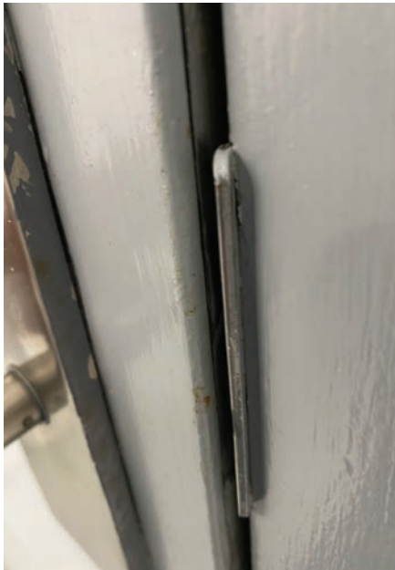
Figure 15. You can see how much play there is in the door.
