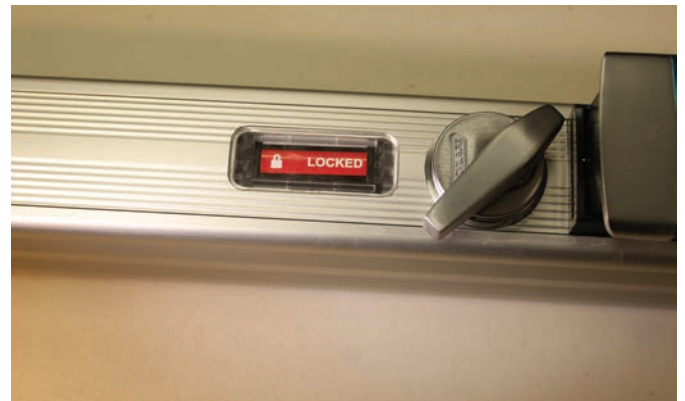
Figure 16. With the device undogged, the indicator shows the device locked. It may sound simple, but always remind your customer that the door needs to be closed and latched for it to truly be locked.
