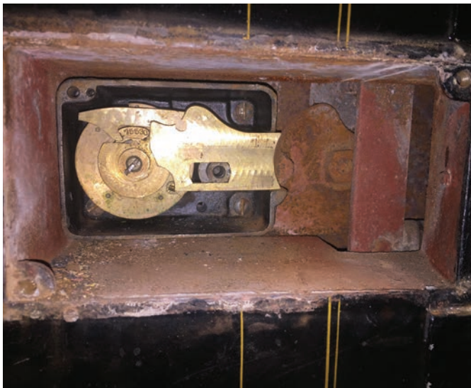
Figure 11. The lock bolt is retracted.
