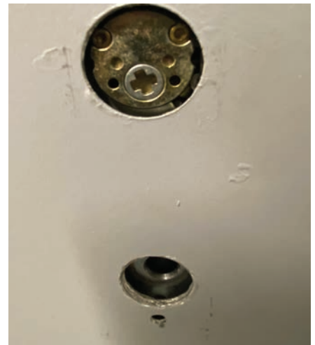
Figure 6. This extra hole left an unnecessary hole on the other side of a fire door.
