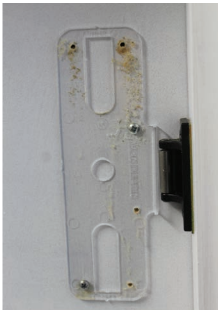
Figure 11. Installing the device on a door begins with installing the strike at the correct height. Then use the plastic template to mark or drill all the mounting screw holes.
