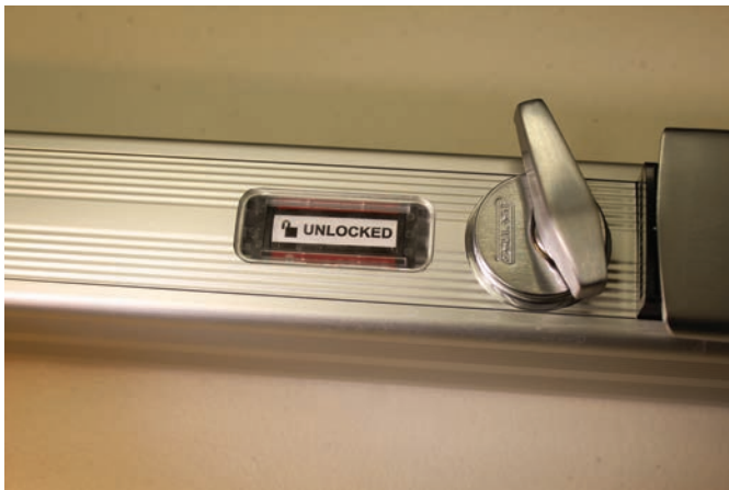
Figure 15. This image provides a close-up view of the indicator with the device dogged down.
