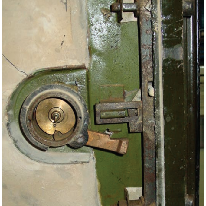
Figure 15. A Yale OB-style lock is shown.
