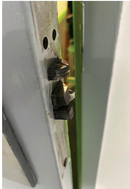
Figure 16. Somebody had decided to grind off part of the latch as well.
