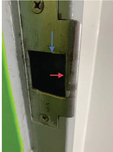
Figure 13. Someone had previously removed almost \frac{1}{2} " of metal (red arrow). The blue arrow points to where the opening used to stop before they removed the metal.
