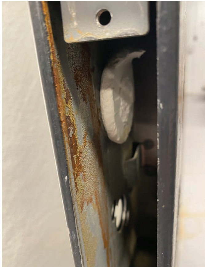
Figure 17. The author looked in the prep and saw this plaster disk.
