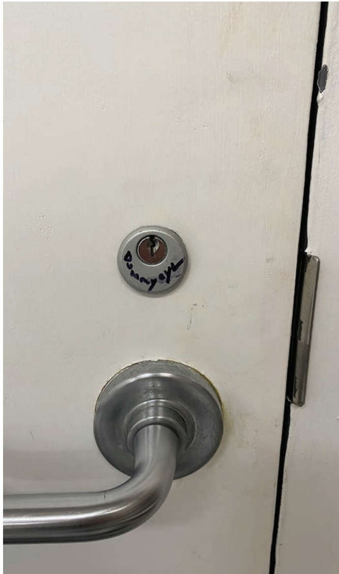
Figure 21. The author had run out of dummy cylinders, so he used a standard cylinder upside down in its place.
