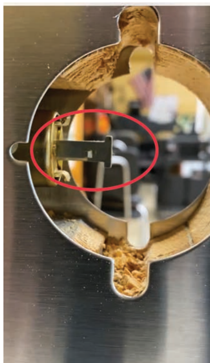
Figure 11. The red circle shows that the latch is still depressed while the door is closed and not in the strike hole.
