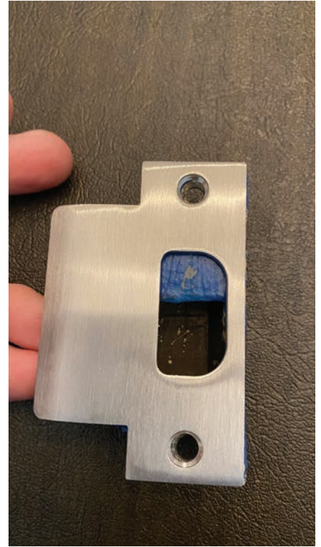
Figure 9. The new strike is on top of the old one so you can see it's an exact fit.
