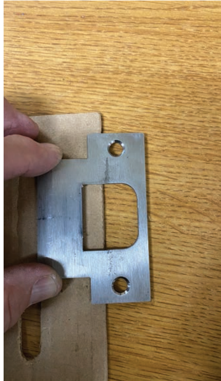
Figure 14. The piece of cardboard roughly represents the metal that had to be removed for the strike to work.
