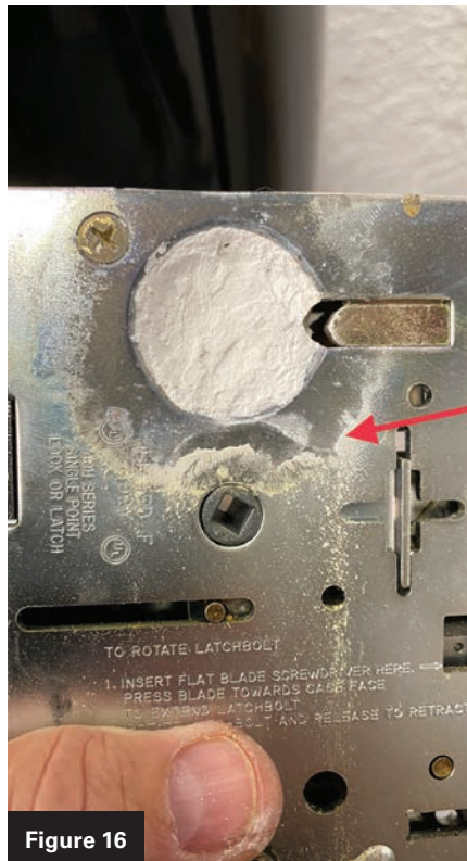
Figures 15 and 16. Notice the discoloration around the plugged cylinder hole.
