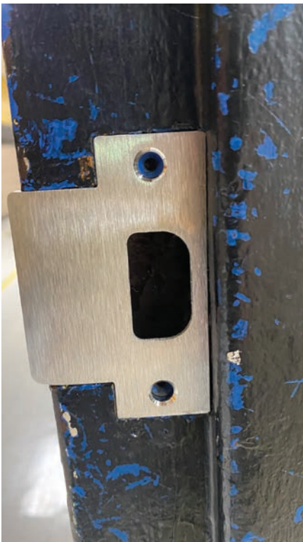
Figure 10. The new strike is in place on the frame.
