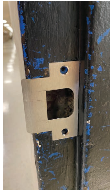
Figure 12. The strike modified so that the latch will drop into the hole.
